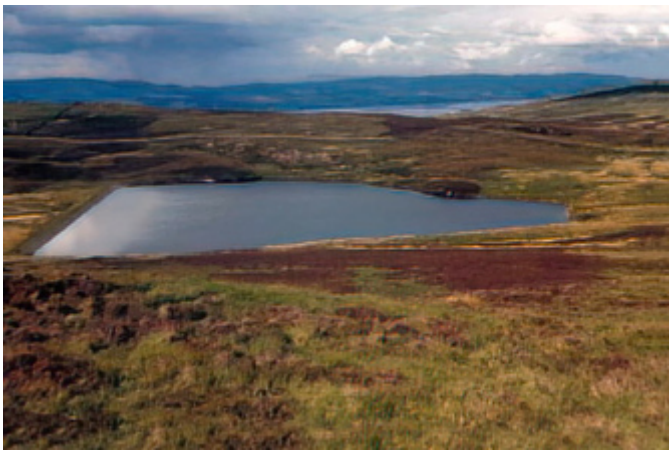
Yetts reservoir From The South
